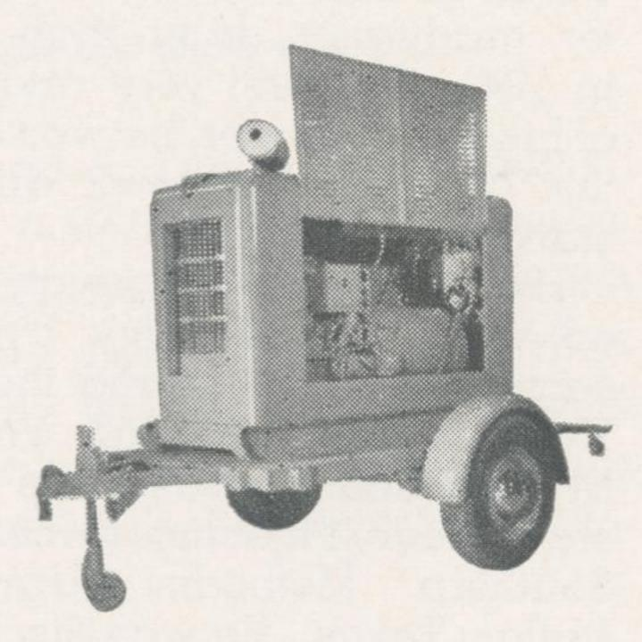
U. S. MOTORS MANUFACTURES STANDBY UNITS UP TO 200 K.W.
