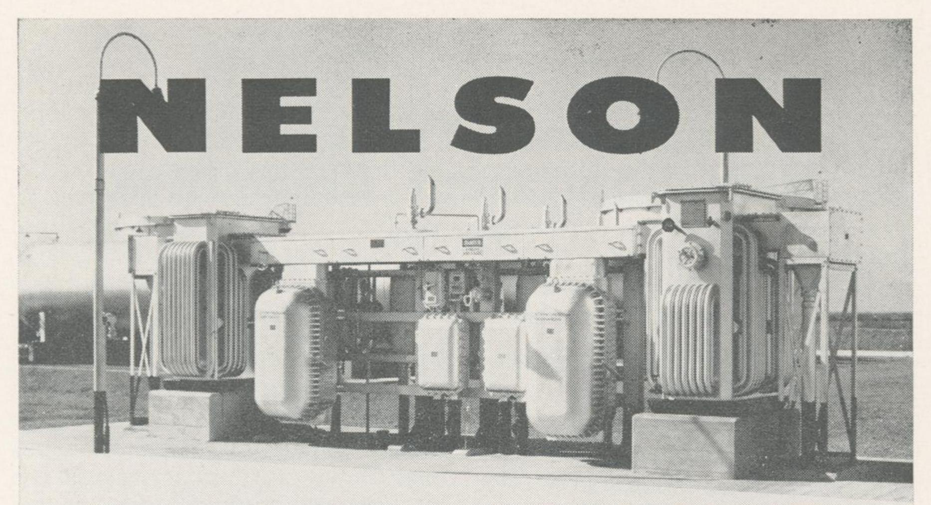
Nelson Class 497 Steel Switchrack with Explosion-Proof Network Protectors, Current Limiters, and Weatherproof Bus Duct installed at a Petroleum Refinery in Class 1, Group D, Division 2, hazardous location.
