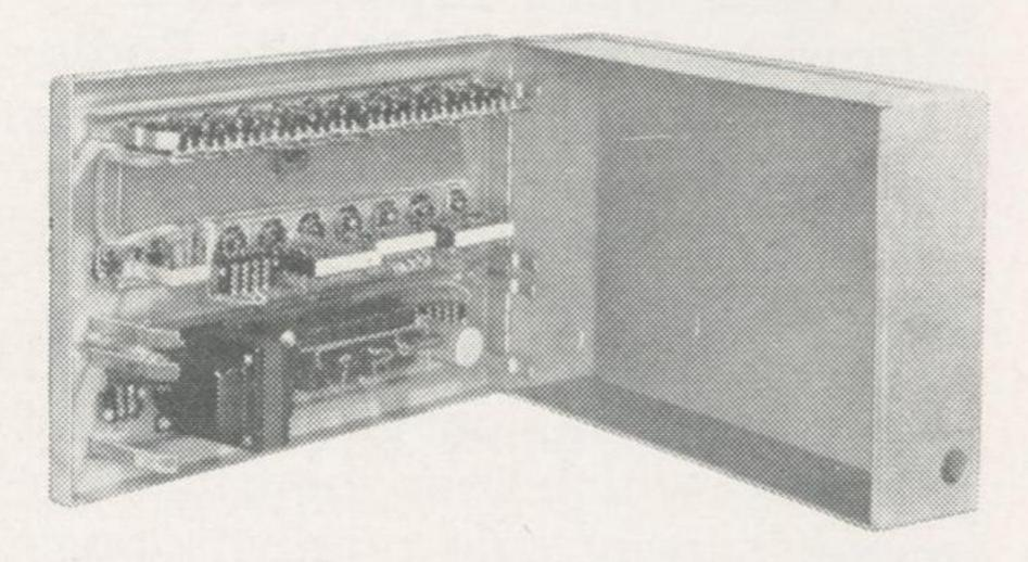
CDX-80RP Relay Panel and CDX-85 Power Supply in wall cabinet. Shown in open position.
